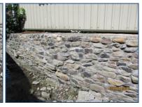
As part of a wide range of measures to reduce the effects of flooding through the centre of Skipton, GallifordTry tasked Ram Services to seal and strengthen a section of drystone retaining wall alongside a watercourse through the town.
